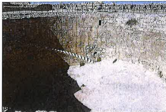
Umayyad water cistern
